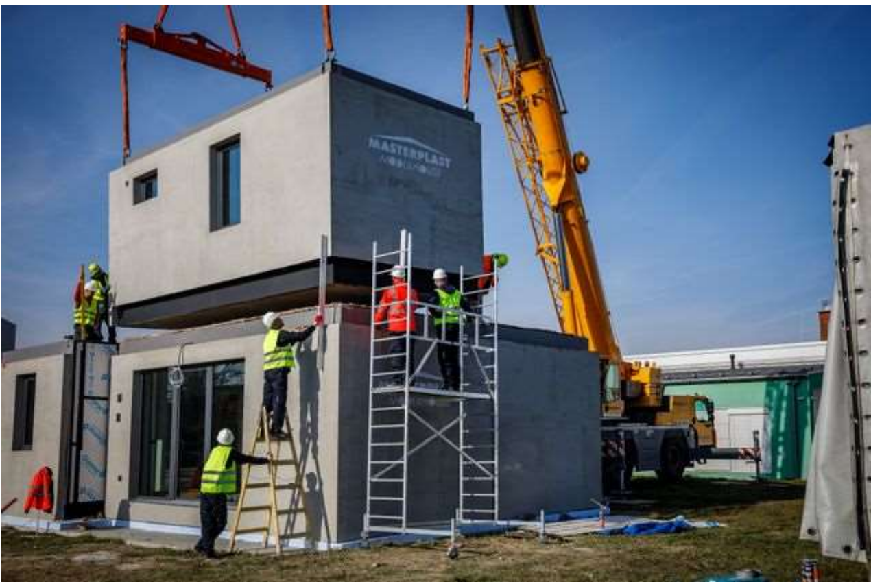
Masterplast Modulhouse construction
